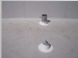
Davit base w/ tieback anchor
