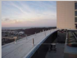
Outrigger supports w/ horizontal safety life line
