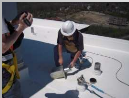
Through slab sleeve w/ portable rigging box
